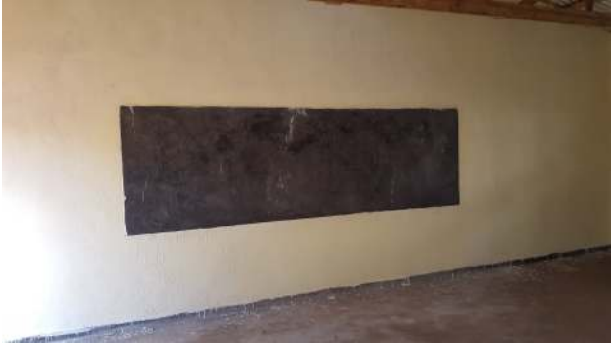
Photos: Blackboards fixed ready for classrooms
